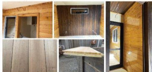
^ L: Linscod oiled interior cypress timber; thermally modified cypress feature wall; entrance porch; thermally modified poplar cladding; engineered eucalypt flooring.
