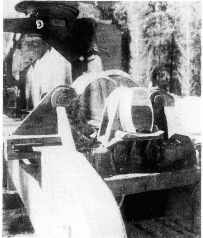
Figure 2: The Hahn Harvester showing the delimber head and knives
