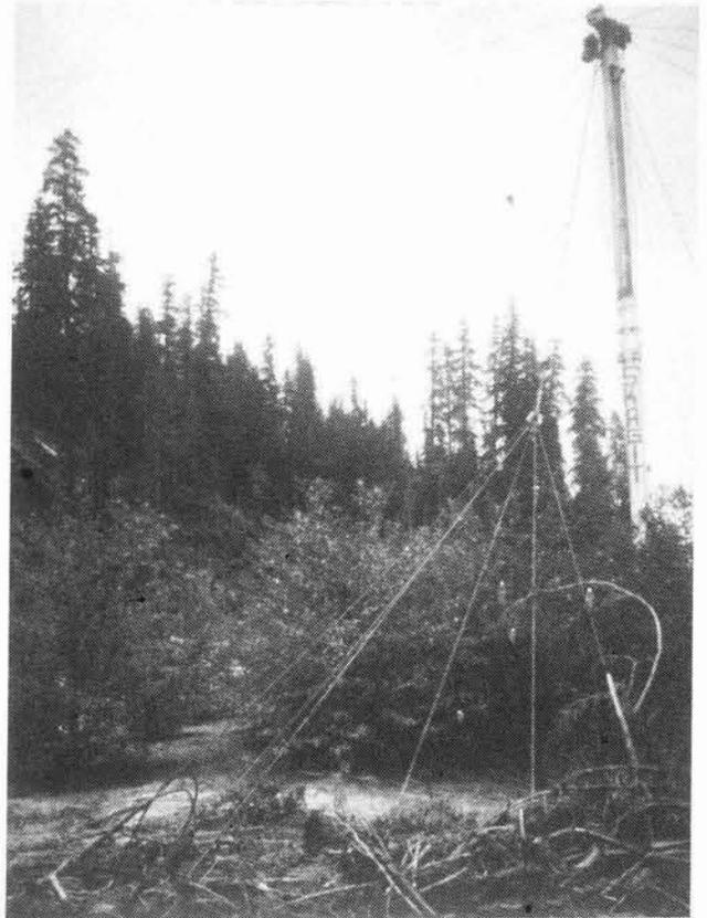
Figure 2- Cluster of six Manta Rays used as a guyline anchor on 34m tower.
