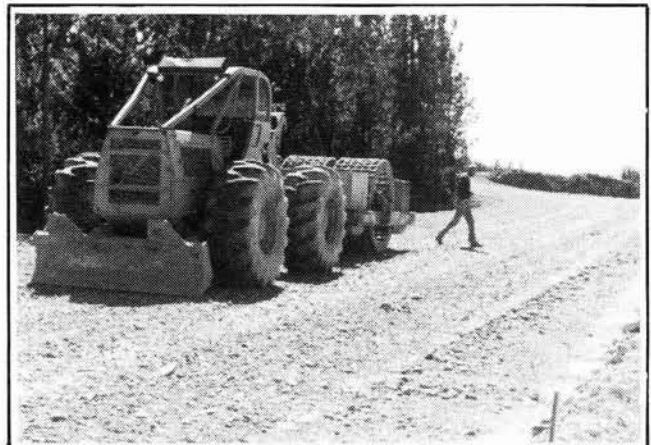
Figure 5 - Grid roller used for base course compaction
