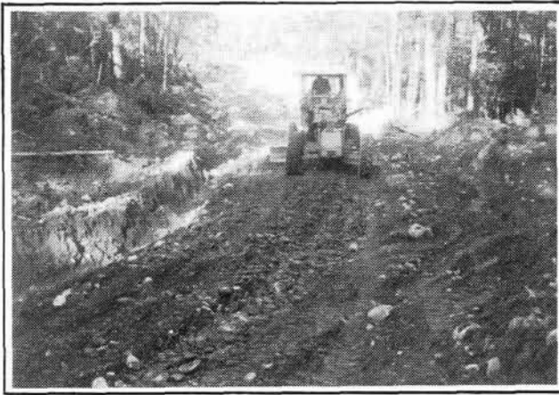
Figure 7 - Constructing a spur road in indigenous forest
