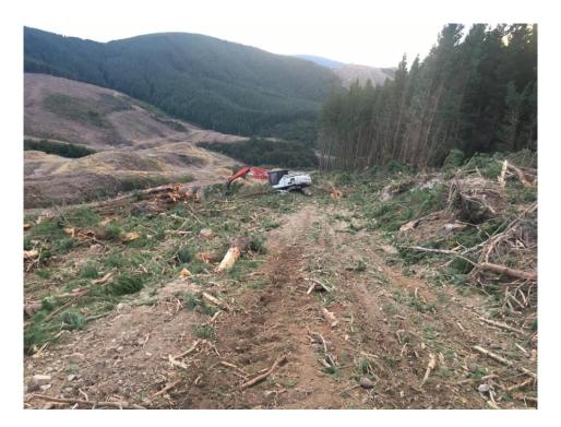
Figure 17: Skid trail Path 1 in operation, leading down to the shovel. The deep disturbance measure was almost exclusively from the main skid trails
