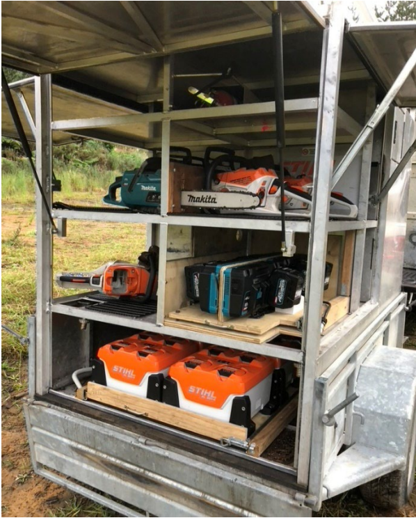
Fig 9: Batteries in the charging facilities, mounted on slide out trays in the trailer.
