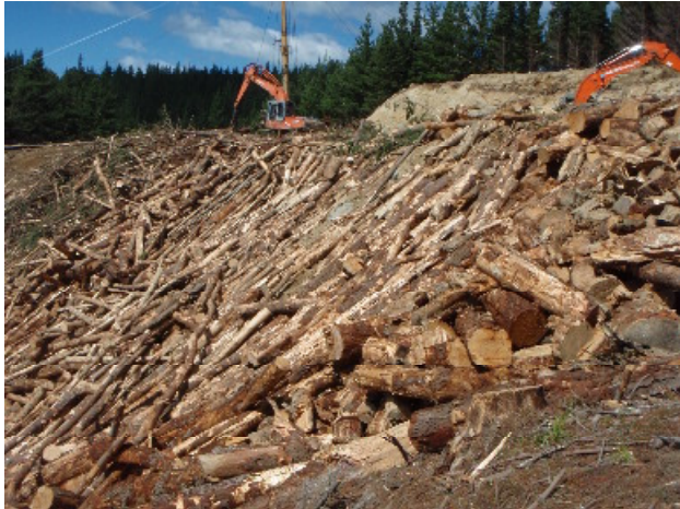
Figure 4. Typical yarder landing showing the biomass discarded 'over the side'
