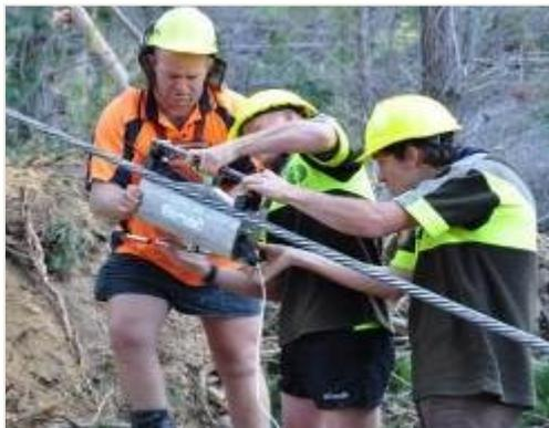
**Figure 8: Mounting the tension monitor on the tethering cable.**
