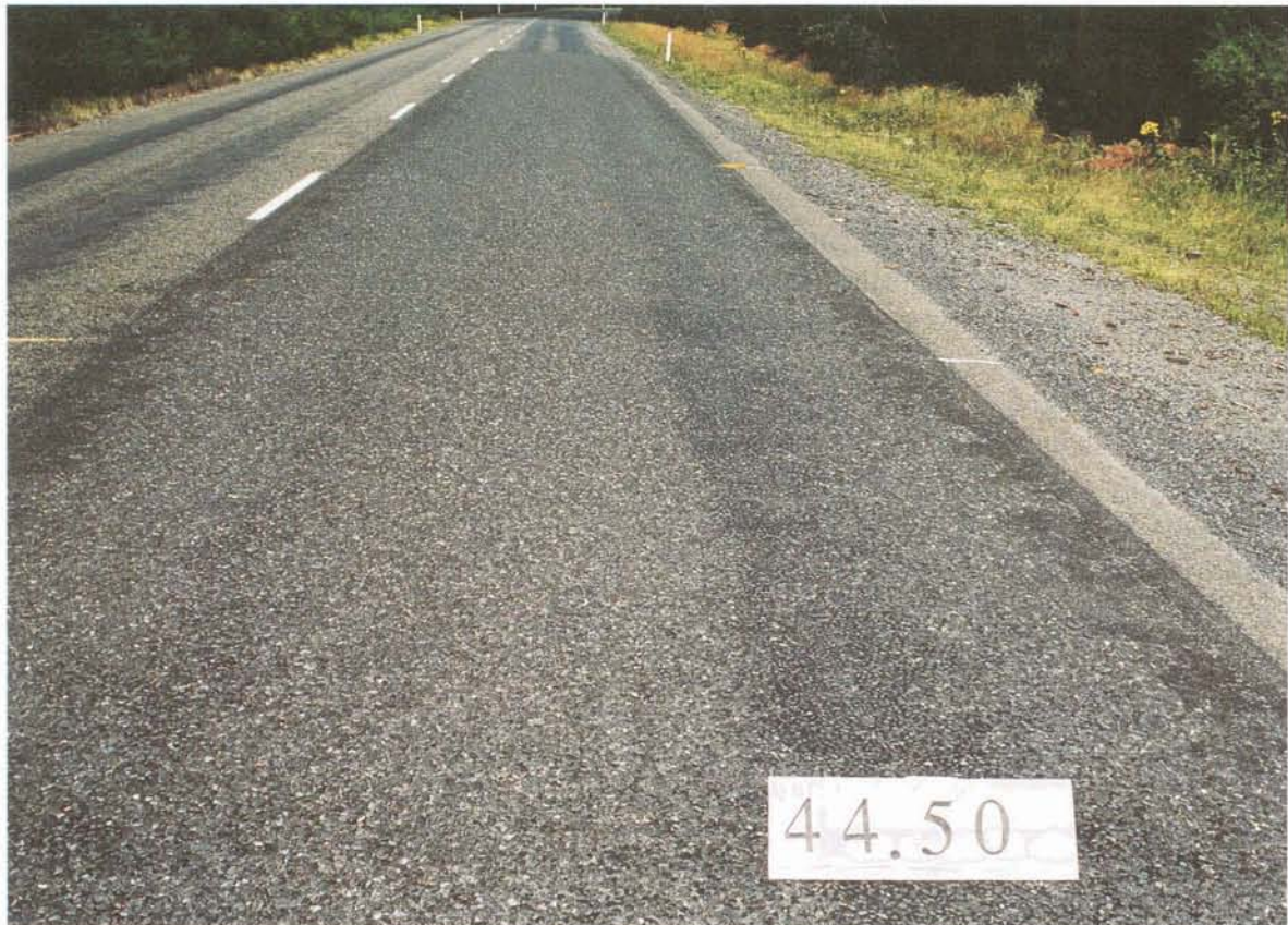
Figure 5 - Chip loss occurring near the centreline and shoulder for the 80/100 section on the flat
