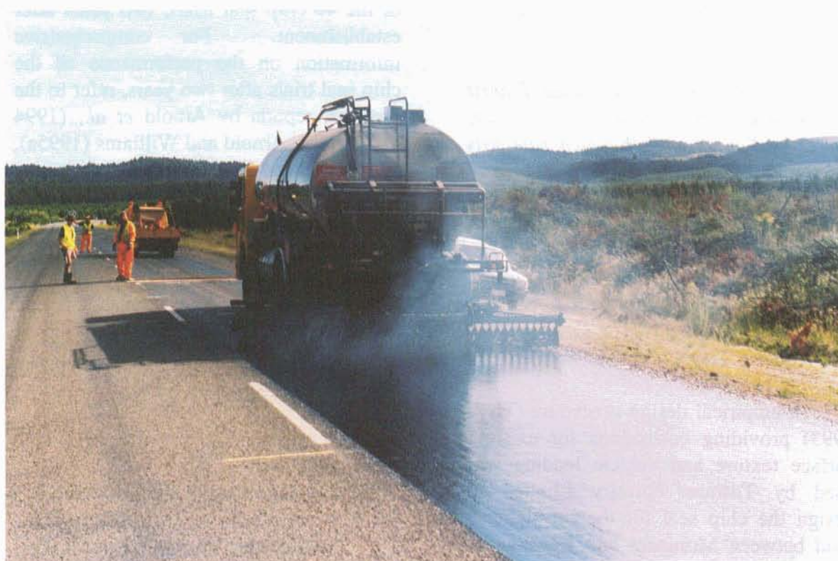
Figure 1 - Construction of chip seal trial sections on Railway Road in Kaingaroa Forest
