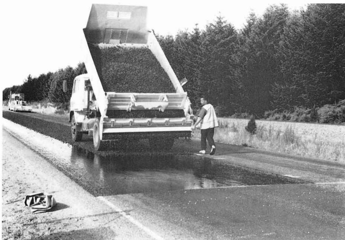
Figure 1 - Construction of chip seal trial sections on Railway Road in Kaingaroa Forest
