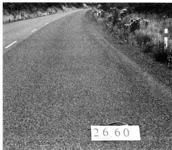
Figure 7 - Chip loss on the shoulder after 12 months
