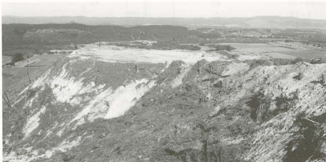
Figure 6 - Bark spread on fill slopes below a landing, Omataroa Forest, to reduce visibility from Rangataiki River plain in the background
