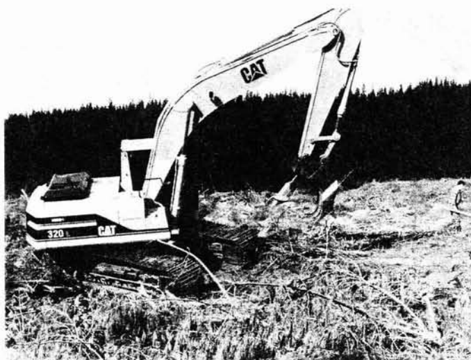
Figure 2 - Excavator with spot ripper-moulder attachment
