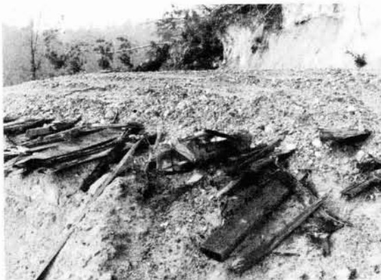
Figure 4 - Mill slabs used as corduroy in Tuatapere
