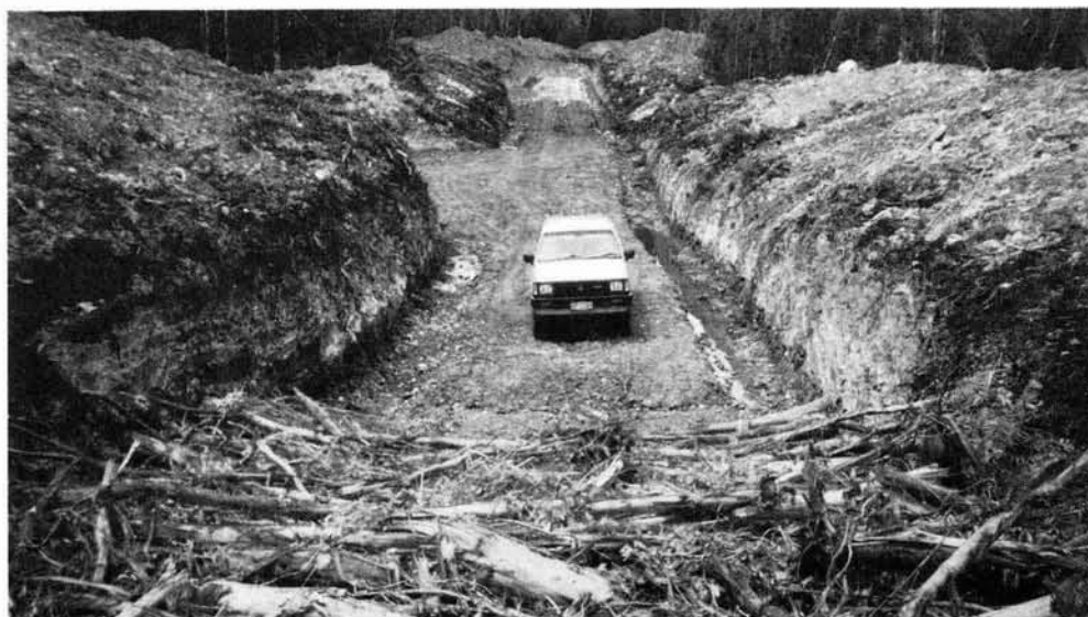
Figure 1 - Rata used for corduroy in an indigenous forest located on the West Coast of the South Island
