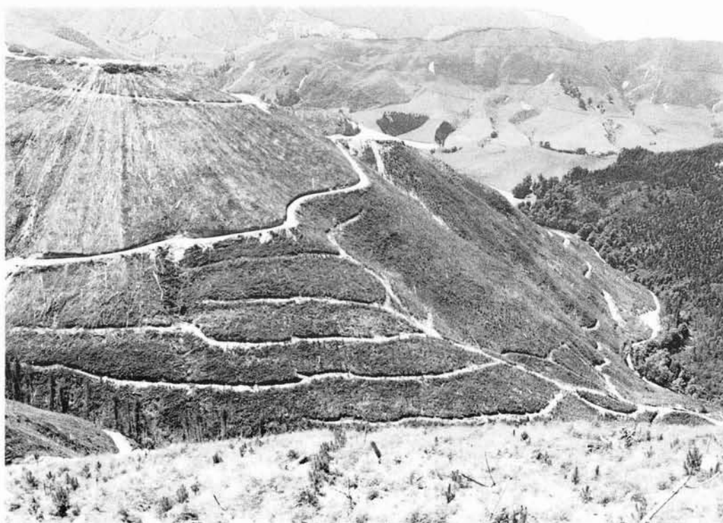
Figure 1 - In steep terrain, erosion from road, track and landing surfaces can be a major contributor to stream sedimentation
