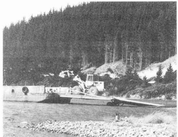
Figure 5 - Barge loading, showing the beach pad, wheelbarrow and shore anchor
