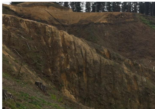
Figure 11: Soil disturbance resulting from poor deflection
