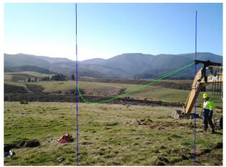
Figure 2: LineSmarts photo processing showing tail hold position and estimated shape of skyline catenary.
