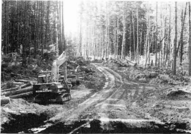
Figure 3 - The Roding Crew Move into Stump and Form the Road
