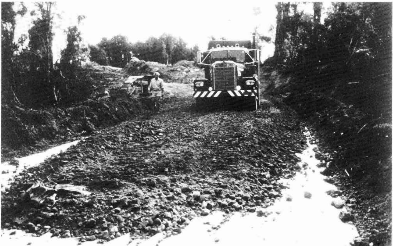
Figure 1 : Geotextile as a separation layer between subgrade and basecourse on a forest road
