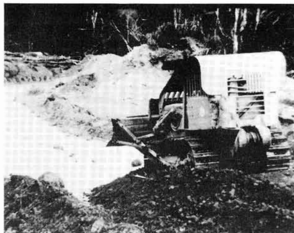
Figure 4 : A good depth of material over a neatly laid geotextile, which is being used as a separation layer between clay and good quality roading material
