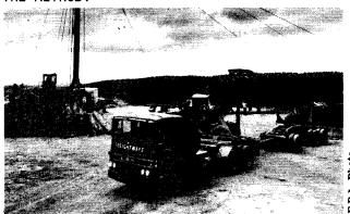
landed tree lengths in front of a Madill spar where they were trimmed and cut-to-length, with chainsaw, by three skiddies. The loader studied, a Fiat-Allis 645-B rubber-tyred front-end log loader, was used to clear the prepared logs from the hauler, sort and stack the required log assortments, and load out logs onto trucks as they arrived. The sorting, stacking, and loading operations were carried out clear of the hauler operation but on the same landing.
