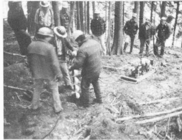
Figure 5 - A 20cm hole is drilled with the Little Beaver auger.
