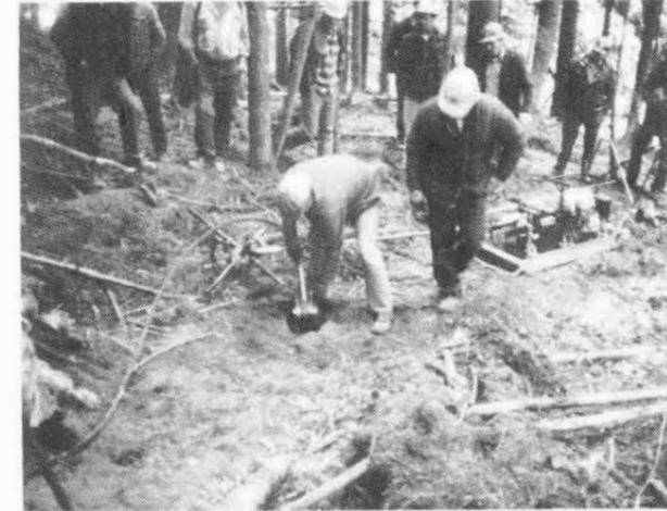
Figure 7 - Lowering a soil toggle into the hole.
