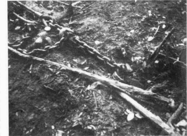
Figure 8 - The chain and hook attached to the soil toggle can be used to equalise the lines in a cluster.
