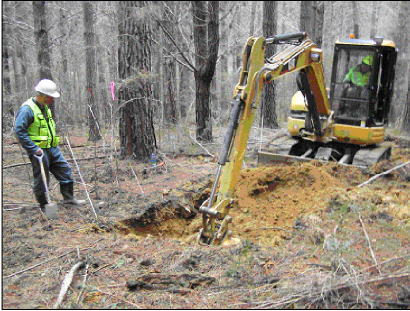
Fig. 2 Excavating a 3.5 m long by about 1.5m deep trench at right angles to the ripping direction.
