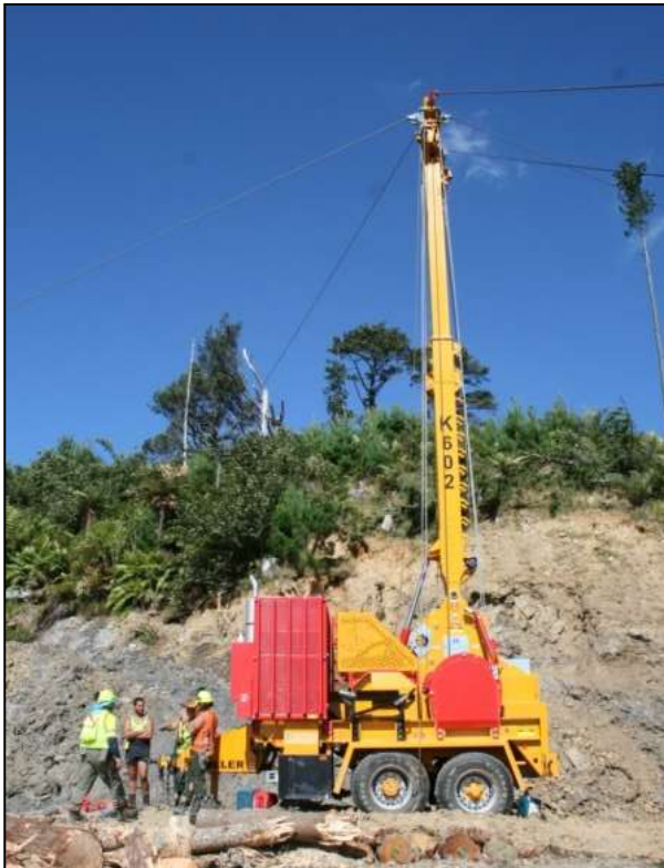
Figure 1: Koller K602H yarder on site
