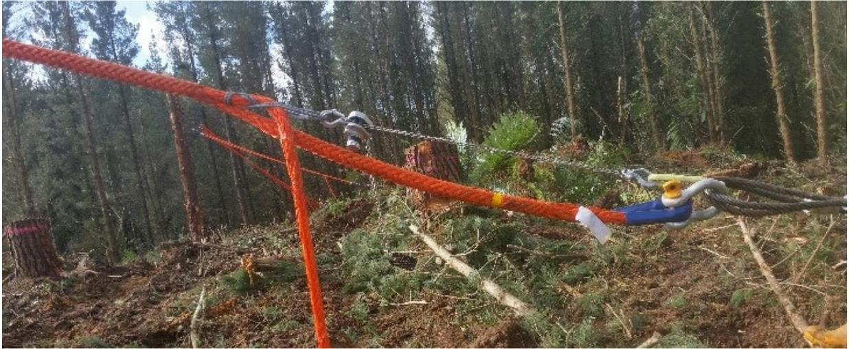
**Figure 15: Tightening the adjustable synthetic guy ropes with a light weight “cumalong”.**
