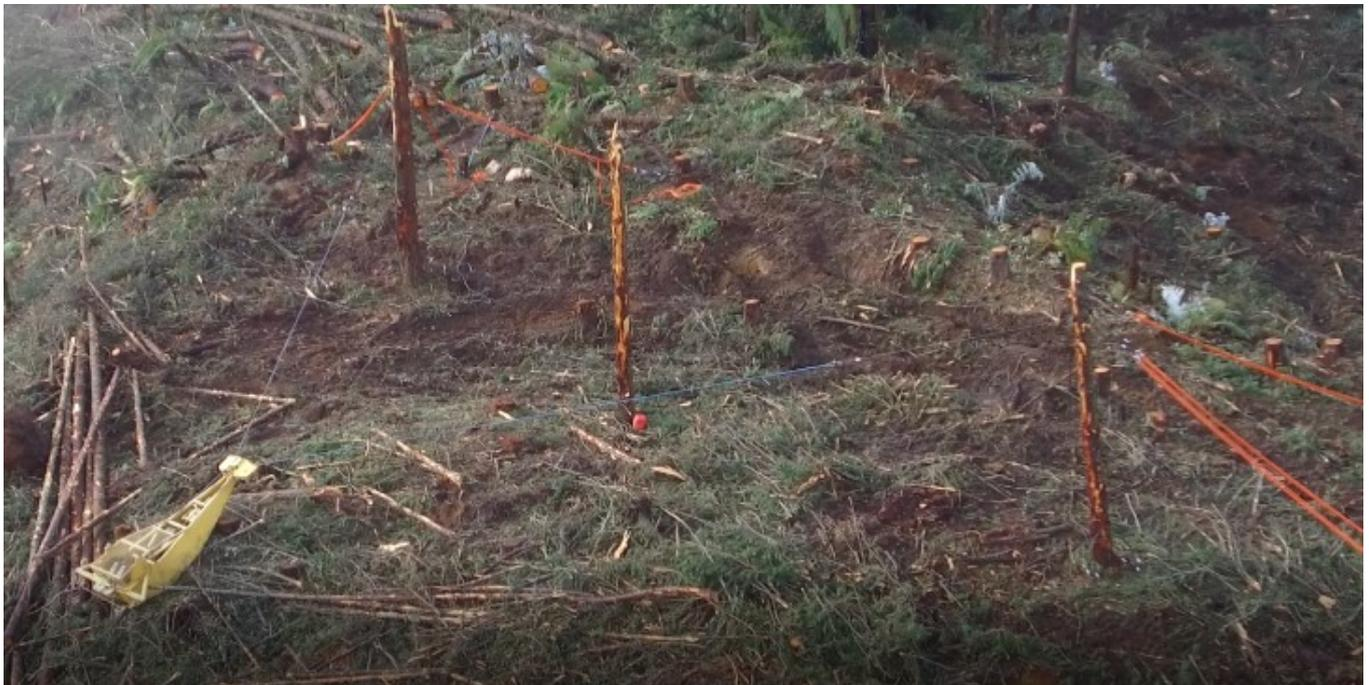
**Figure 12: Elevated anchors ensure Skyshifter and winch ropes can be lifted clear of the ground.**
