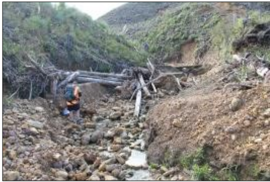
Experimental weir near road completely filled with sediment. Note the riparian failure upstream, and woody debris in channel.
