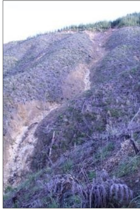
Upper-slope landslide arising from a roadside fill slope and subsequent debris flow track scouring tributary channel to bedrock and delivering material directly to stream.
