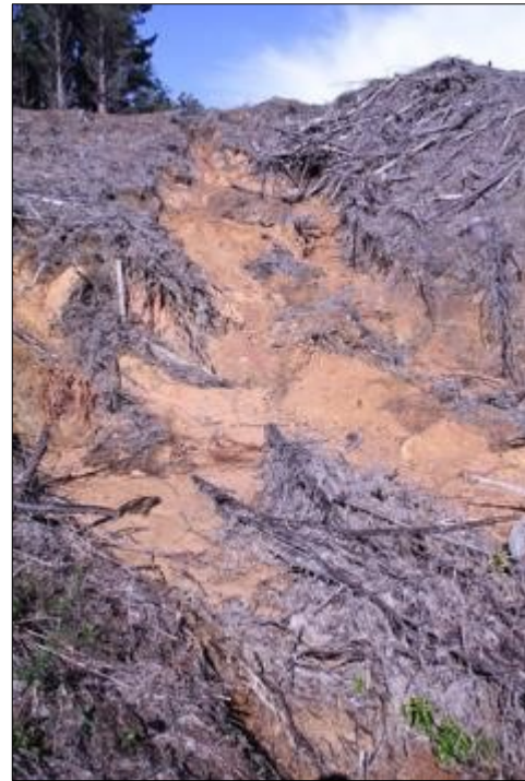
Failure below or from a landing. Material ended up in valley floor. Directly opposite the photo on left.
