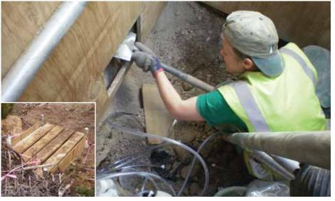
Amanda Matson installing lysimeters in a soil pit and completed pit directly after fertiliser application (inset).
