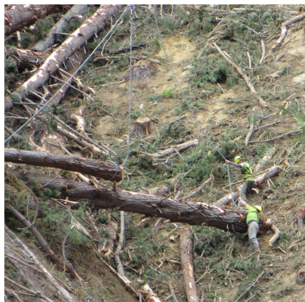
Figure 1: Breaking out on steep terrain
