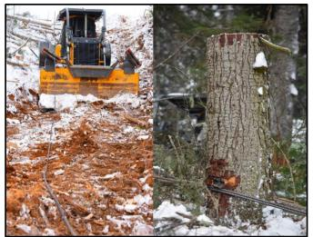
Figure 37. Example of a catch tree being used at Case Study 6
