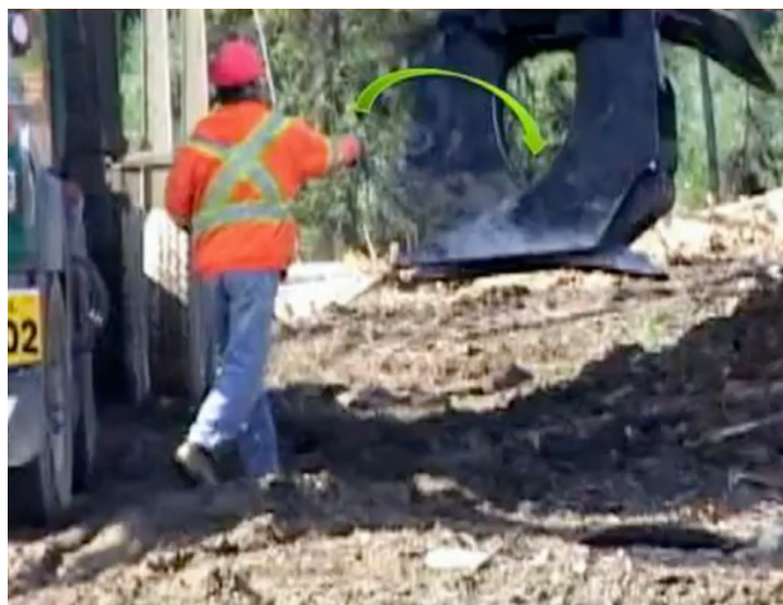
Figure 6. Excavator assisted chain throwing using a grapple loader (FPIinnovations, 2021)
