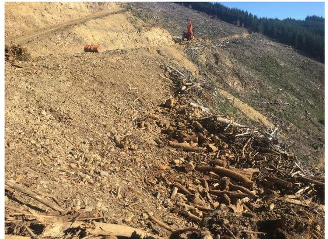
**Figure 7: Harvest residues that were covering this slope below a landing have been extensively pulled back as part of the Azwood recovery operation.**
