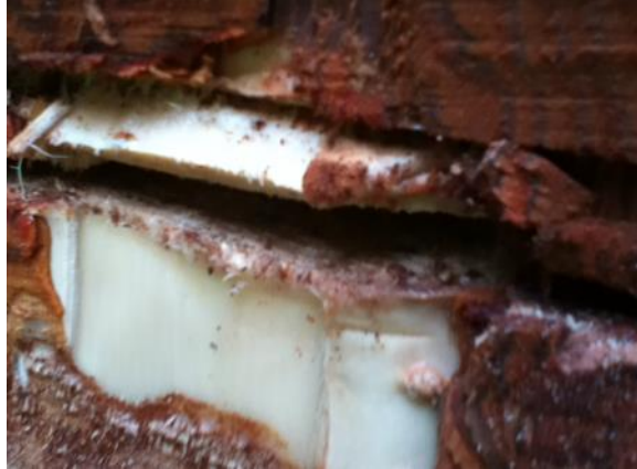
Figure 13: Result of Koller wedge forcing itself out of the back cut
