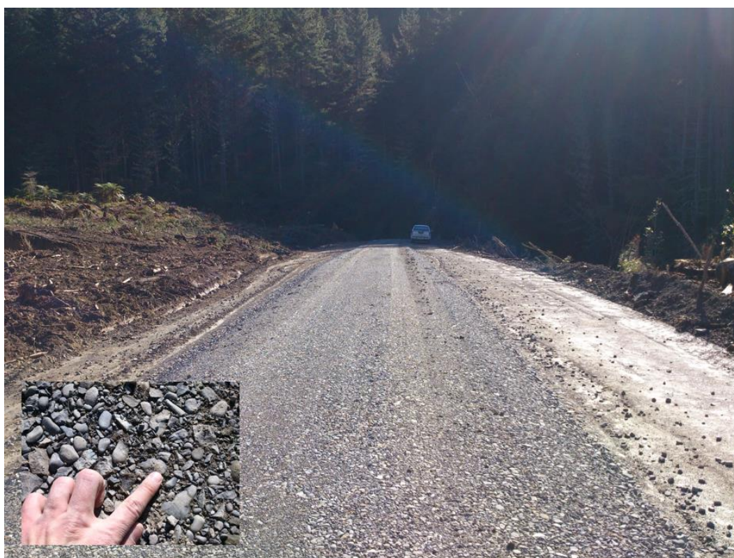
Figure 3. Newly-constructed secondary road on the East Coast.
