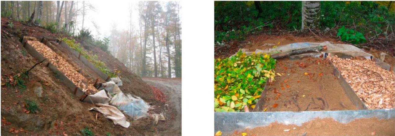
Figure 2. The setup to collect runoff from different surface cover plots of woodchip, slash and a bare control plot (Turk, 2018).
