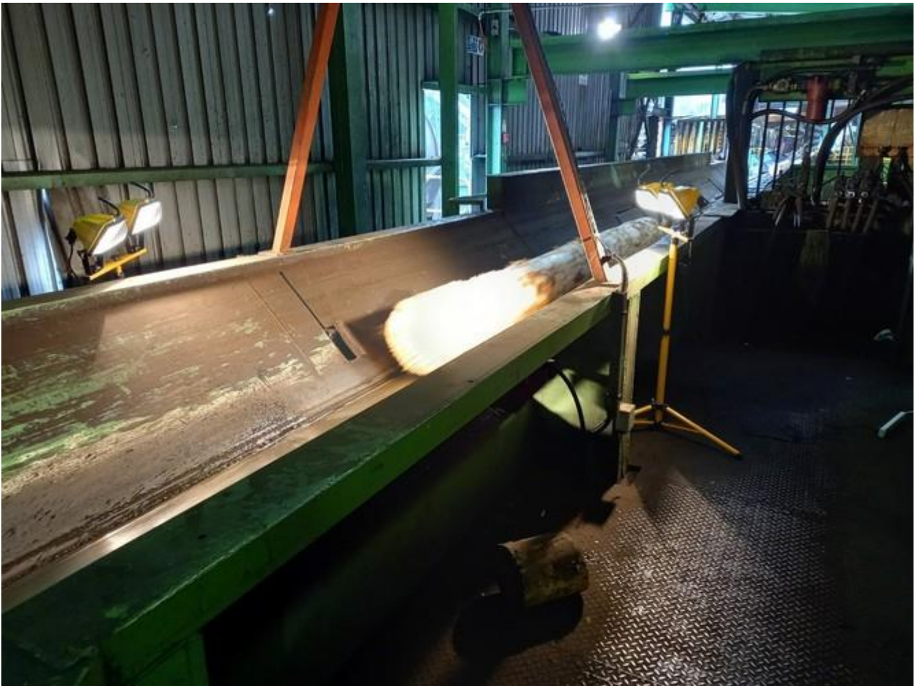
Figure 2: Installation of the lighting.
